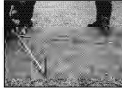
**3** Establish the position of your last corner point. Repeat Step 2 to locate the last corner point. Measure the length of the fourth side and use the length of the diagonal to test it. Hammer the last peg into the ground.
