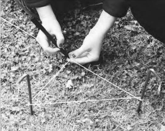
Even after you've strung out your trench, it's possible for the string to move (or, more likely, for some unfortunate person to trip over it or kick the pegs out of alignment). To make it easier to reconstruct the precise location of your original corners, mark the place where the strings cross with a permanent, easily visible pen line. In this way, if the string is ever moved, you'll be able to see its original position easily and replace it accordingly.
