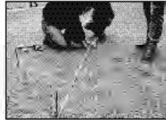
**4** Check your accuracy. Measure the lengths of all sides again and check the length of both diagonals again. Adjust the position of any corner pegs necessary until you have the trench completely square.
