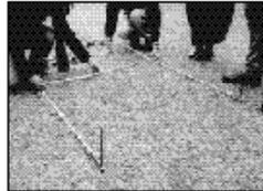
**5** Set up an outer framework of pegs. Place two pegs slightly behind each corner point along the same axes as the sides. These are the pegs that you will actually use to string out the trench.
